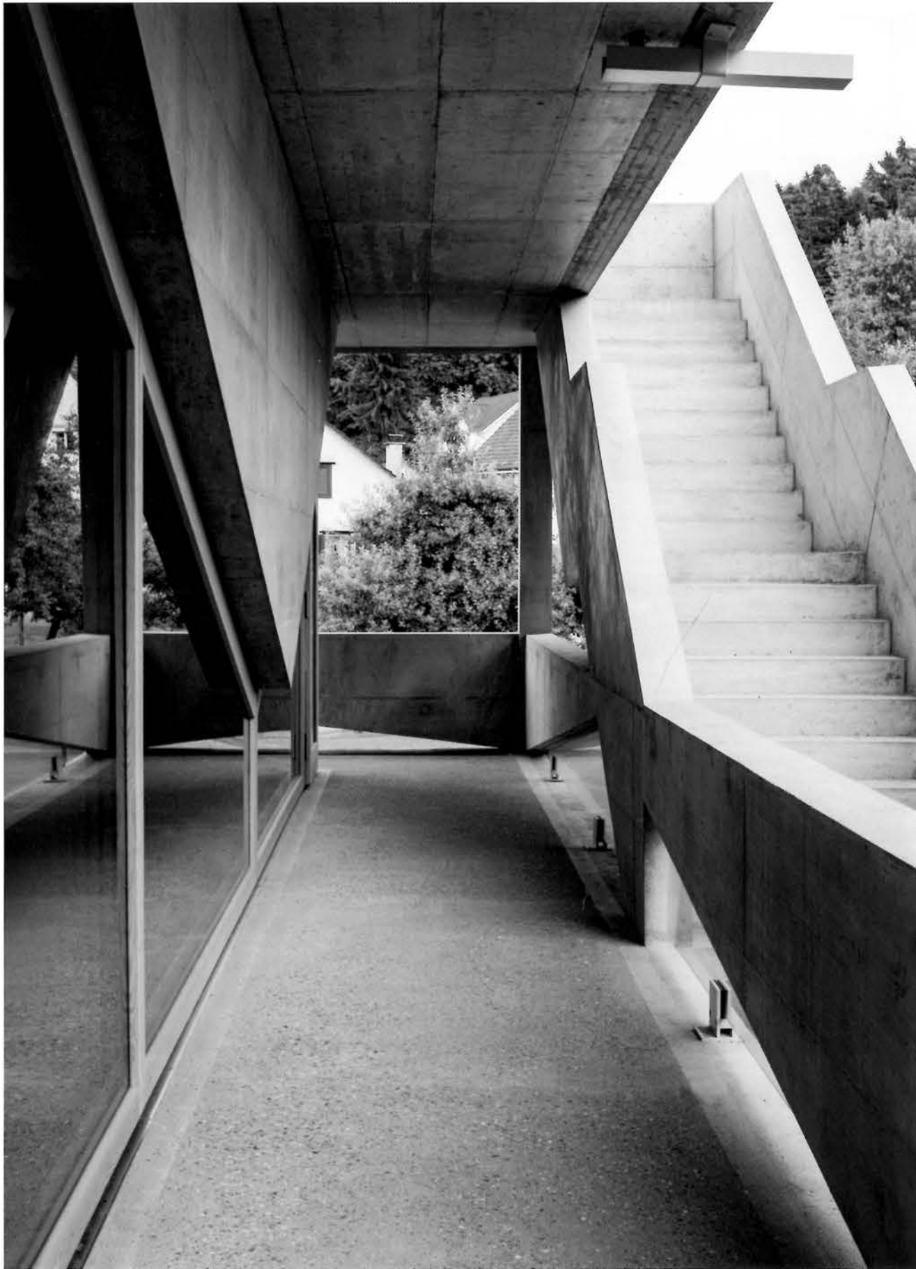
p. 14, p. 15, both images: Two different systems alternate in the definition of the facades, the balcony that runs along the perimeter of the building defines a filter space with its own external mesh, while the internal front is marked by the alternation of large triangular elements that sit on the low columns. This page: View of the sculptural escape staircase located along the corner of the building from the balcony.
